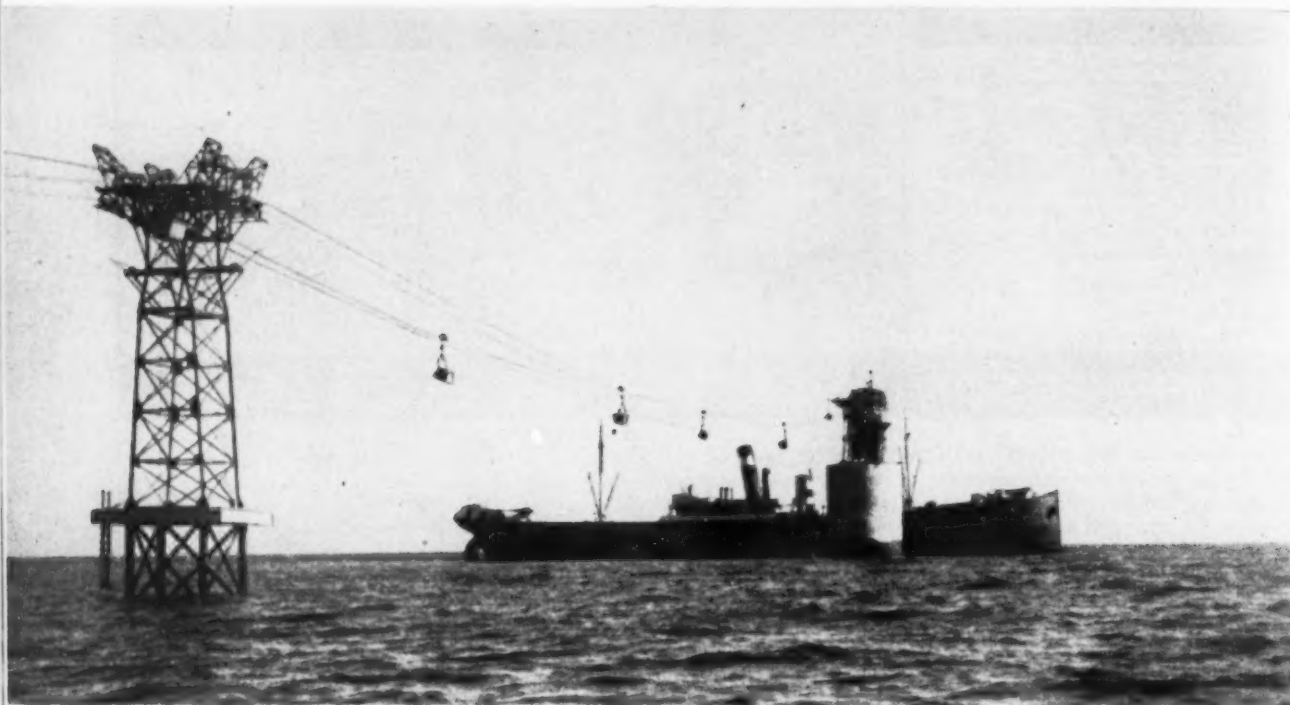
The tramway in operation loading a ship with pyrite.
